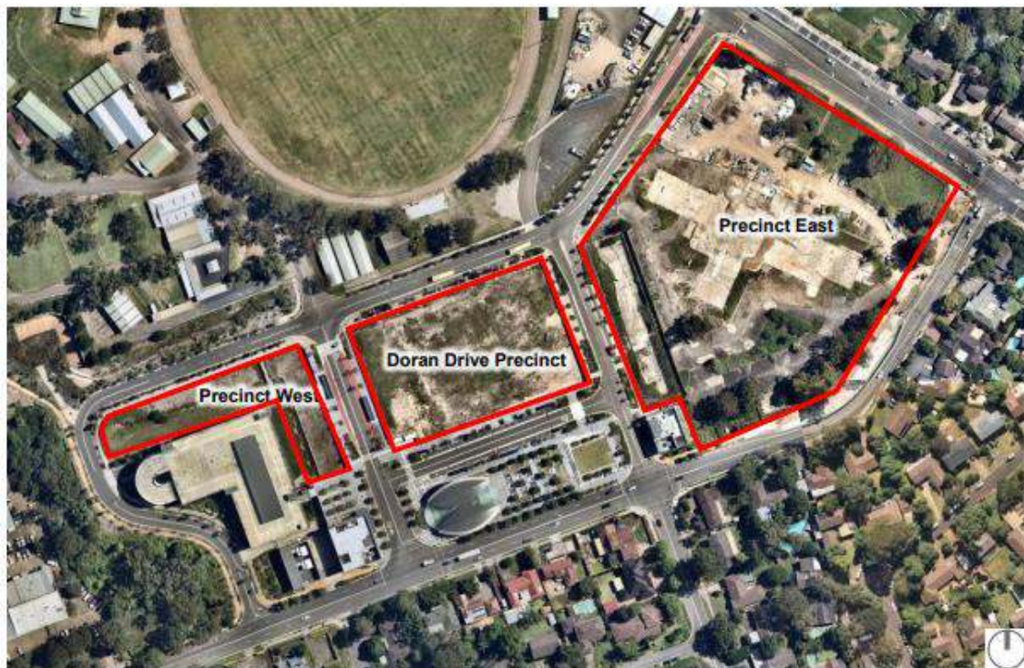
Figure 2: Doran Drive Precinct Site Location (centre) prior to development, Source: Nearmap 2022 / DPE Modification Assessment, 2022
